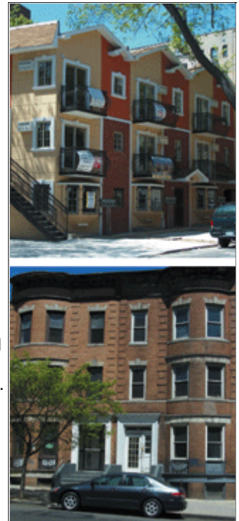
Three-family homes at 366-372 East 201st St. are under construction, top. Two apartment buildings, at 245 and 247 Bedford Park Blvd., bottom, sold this winter for $424,000 each.
